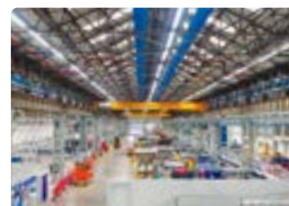
Rolls-Royce – production hall refurb
