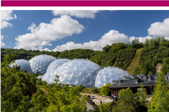
Eden Project 140 kWp roof-mounted solar PV system on plant and education facility
